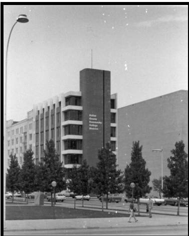
701 Elm Street Assigned to El Centro College when District Office moved to Lamar Street in 2009
